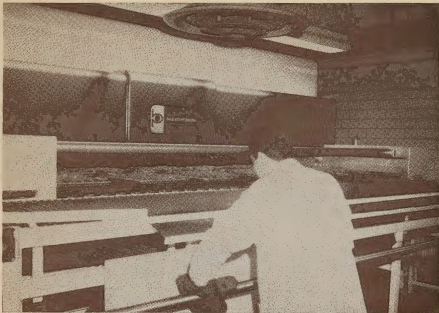
The balls of dough are moved along a conveyor belt. It is flattened and rolled into long cylindrical units. They are then dropped into pans automatically.
